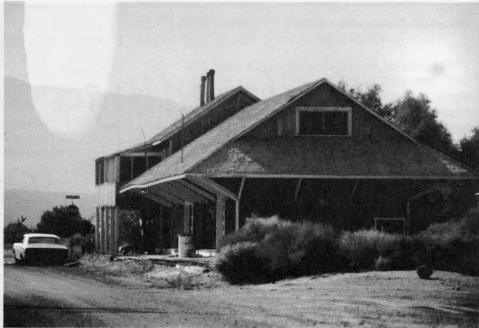
Above: The Carson & Colorado Depot at KEELER was converted into a private home shortly after abandonment by Southern Pacific
