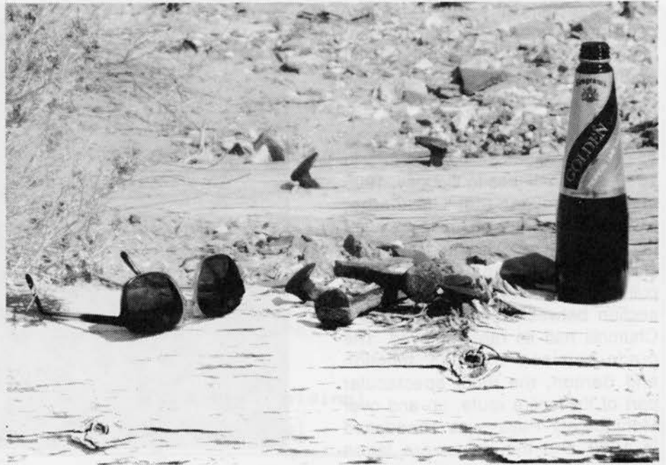
Right: Ties and spikes still lie on the ground on part of the MOCK SPUR, which branched off the main line a few yards north of the present junction of Hwy. 136 and Dolomite Loop Road. Glasses and a bit of refreshment provide scale. March 1988.
