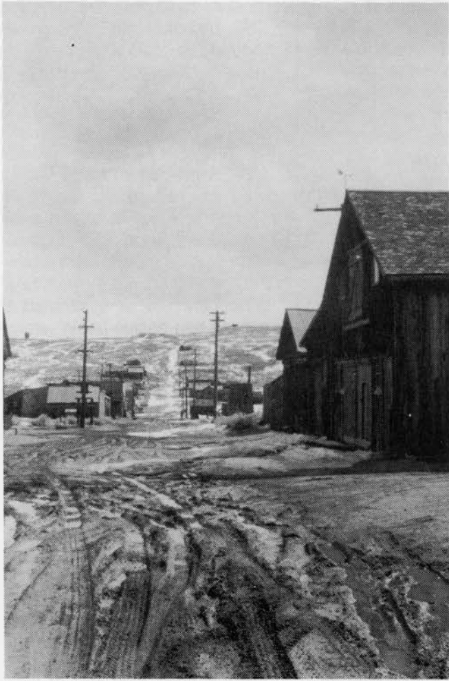
Green Street, Bodie, showing power poles and tree-less hills.
