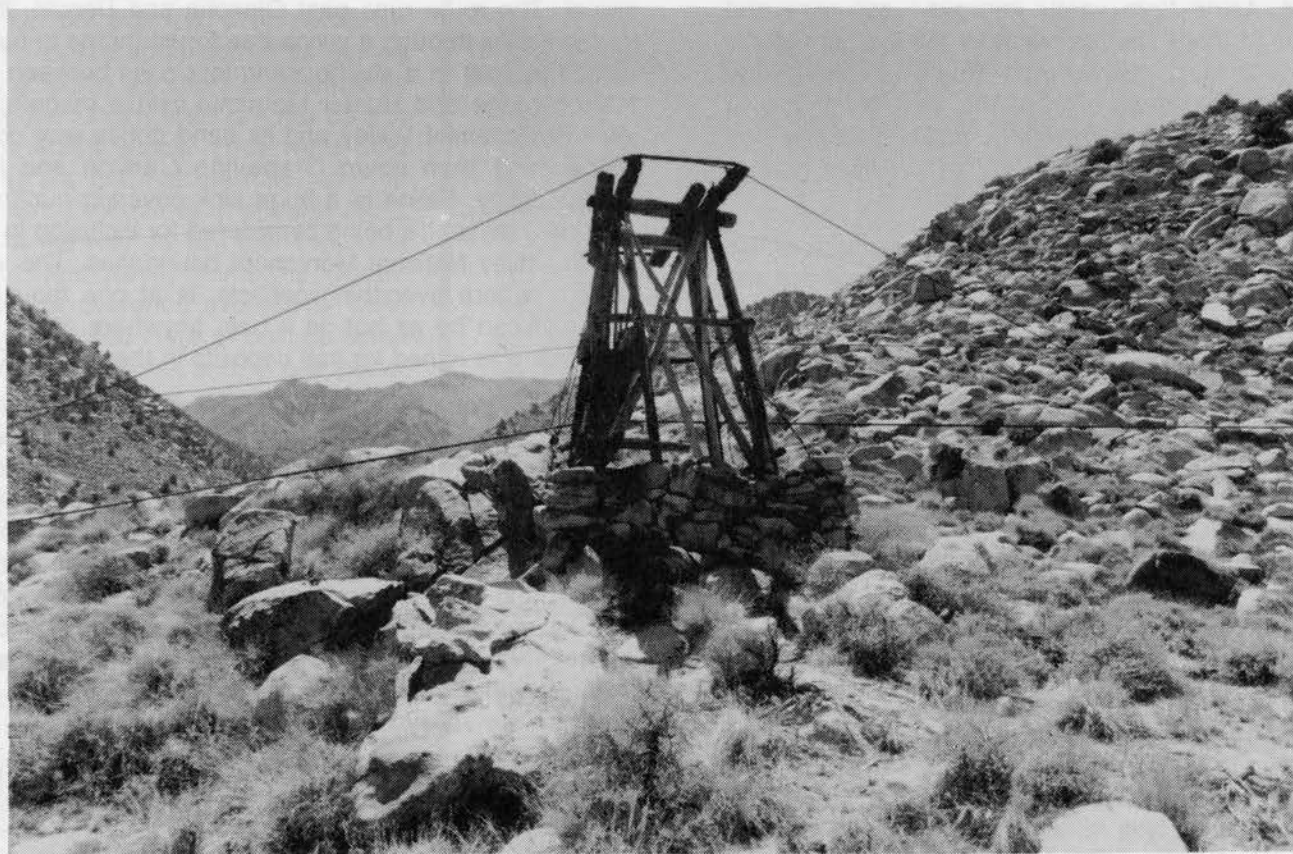
Tram tower above Beveridge. The tram started at the mine 800 feet above Beveridge and ended at the bottom of Beveridge Canyon. Most of the timbers in this tower are of native pinon from higher elevations.
