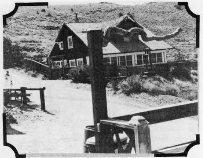
For an extended time windowless and home to only mice and memories, the Gordon House has again become headquarters; this time for the restoration effort.
